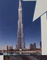
Construction of Burj Khalifa- Luca
